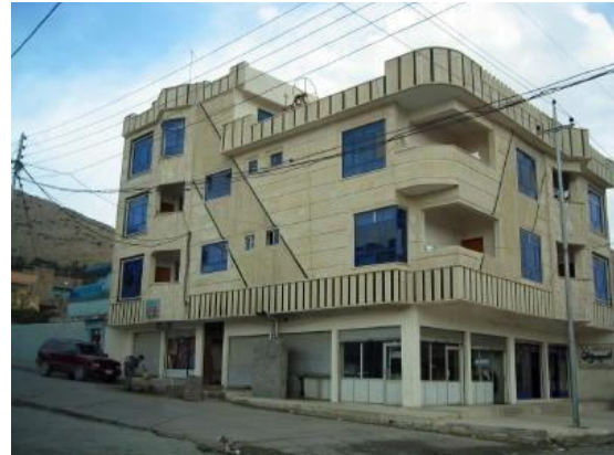
Sample intact building condition image
